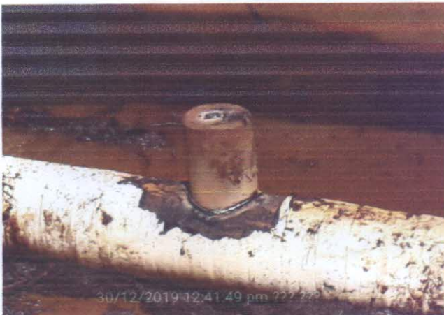
Pic 3. Repair work
